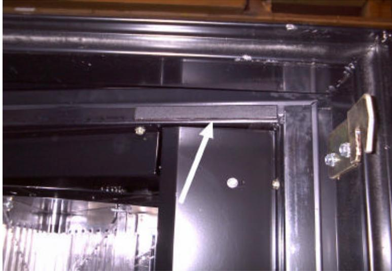
**Attach Magnetic Gauge on the top of the mating strip as shown. This photograph displays magnetic strip attached for the right mating surface; the left side is attached in the same manner.**
